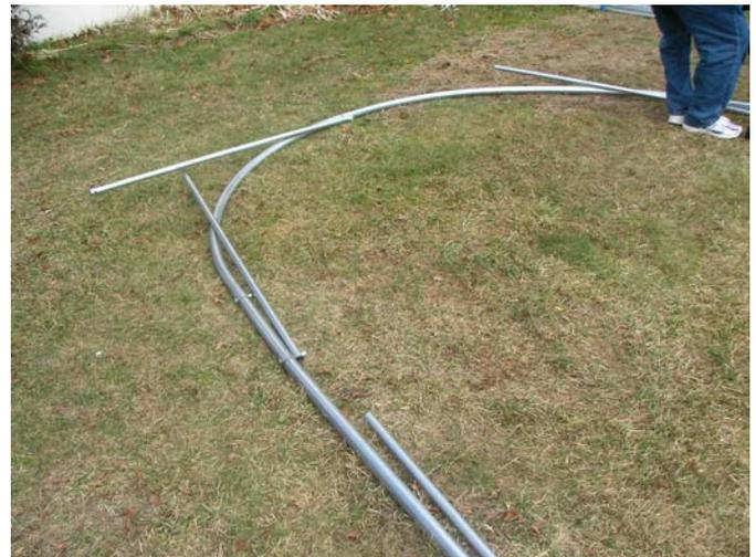
With the assistance of a second person, support the End Arch Assembly vertically. Next stand an interior arch assembly up vertically into position, approximately 60" apart. Connect the Base and Side Cross Rails from the End Arch to the Interior Arch. Align the holes near the end of the cross rails with the holes in the interior arch.
