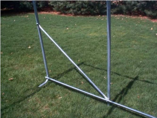
**Step 5.** Begin the Top Ridge Rail by placing the final ECR-2031 Plain End Cross Rail underneath the End Arch Tube. Secure the Cross Rail loosely with a Carriage Bolt CBN-3005-3 with washer and nut facing the interior of the unit. This begins the Top Ridge Rail. The other end of the Cross Rail goes on to of the Interior Arch as shown in the illustration above.
