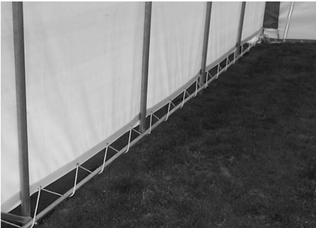
**Step 4.** Retighten or readjust the turnbuckles on both the cover and end panels as needed. Retighten the rope holding the main cover to the bottom cross rail. **Both the cover and the end panels should be checked and tightened on a monthly basis.**
