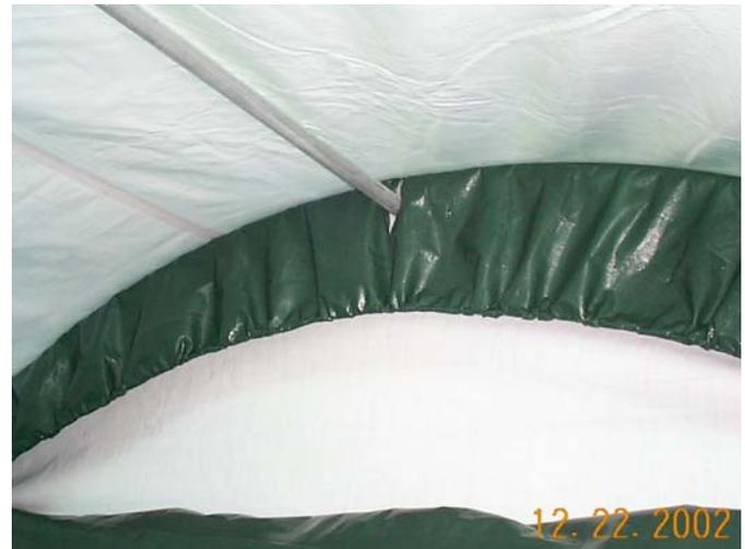
The rope slot should be located inside the unit, with the frame members passing through the pre-cut slots in the end panel/door. Replace the carriage bolts after putting the end panels into position.
