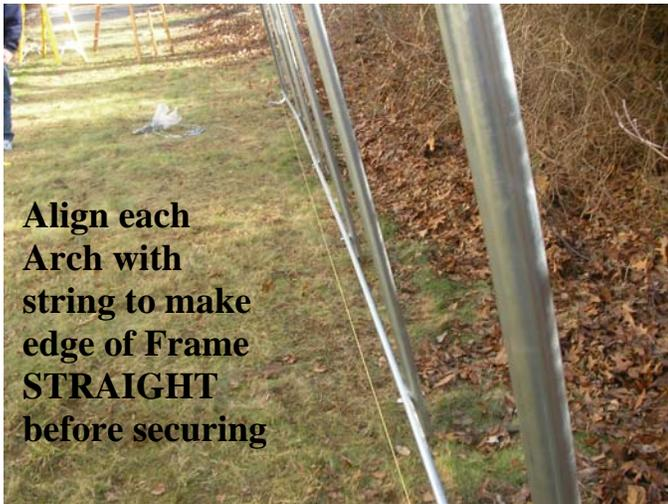
**Align each Arch with string to make edge of Frame STRAIGHT before securing**
