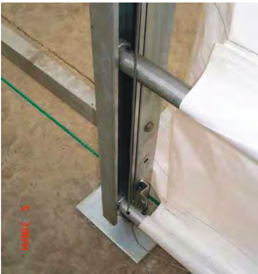
Door Tubes Inserted Into Door Track
