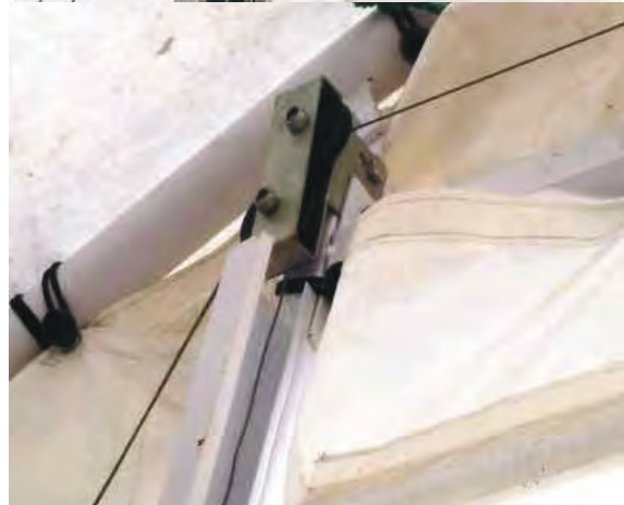
Double Pulley Nearest Winch Assembly
