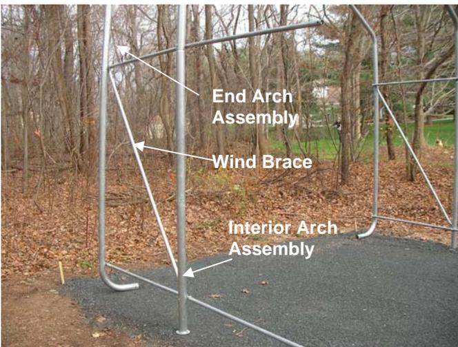
Begin the Top Ridge Cross Rail by placing a #5 Cross Rail underneath the End Arch Top Crest Tube. Secure the Cross Rail loosely with a 3" Carriage Bolt with washer and nut facing the interior of the unit. Male End of next Cross Rail fits into Female end of cross rail. Cross Rails are built by placing rails into each other on the same carriage bolt.
