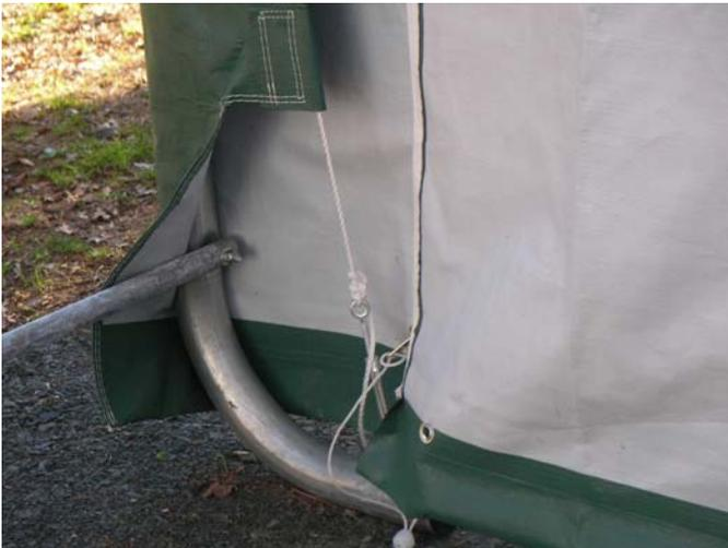
Door Turnbuckle Attached to Base Foot
