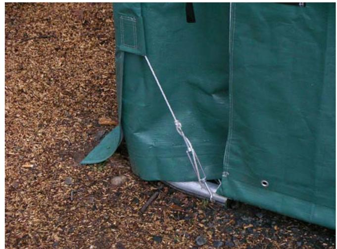
*Main Cover Turnbuckle secured to Base Foot*
