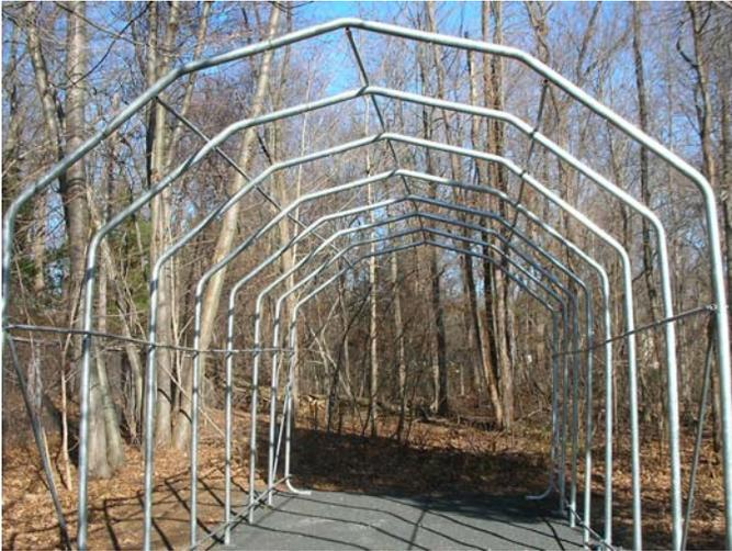
Measure frame width across from outside to outside of frame members. Adjust to 12' width along entire frame length.
