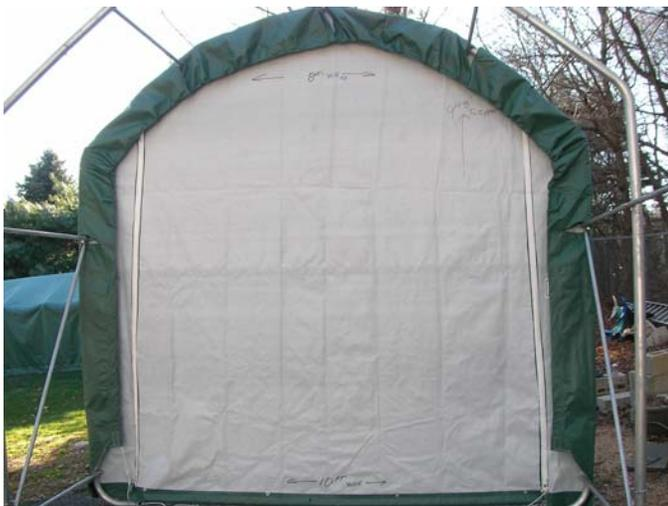
**Note:** After door panel is installed with all slack out of rope, adjust/snug the end panel by turning the turnbuckles or repeating step 3 on a regular basis
