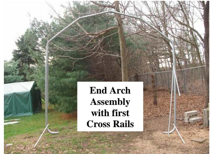
**Step 2.** Assemble the (2) Corner Wind Braces #8 to #2 End Upright w/Foot to the first of the End Arch assemblies. Use a #11 3" Bolt with Washer and Nut to secure the braces loosely to the Upright. Do not tighten completely.
