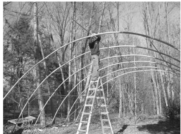
Interior Arch Assembly #5 and #6 have plain feet ends. The last Arch #7 will be the remaining End Arch Assembly with feet. Make certain to install the Wind Braces between the End Arch Assembly (#7) and the
