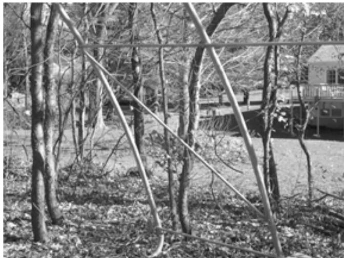
Stand an Interior Arch Assembly (without feet) assembly into place about 60" from end arch assembly. Align holes in Arch with Cross Rails. Using 4" Carriage Bolts, with nuts and washers connect the Side Cross Rails between the arches. Connect Wind Brace from End Arch Assembly To first Interior Arch. This will make the first two arches self-supporting. Insert next Cross Rail into the base and Side Rails for the next arch assembly.
