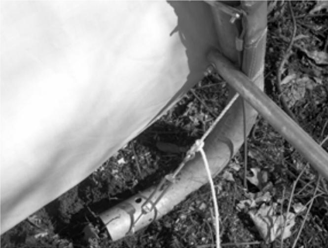
Tie off that end of the rope to a turnbuckle (fully opened) attached to that Corner Foot. The End Panel / Door can then be tightened further by adjusting the Turnbuckles.
