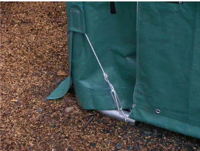
*Main Cover Turnbuckle secured to Base Foot*
