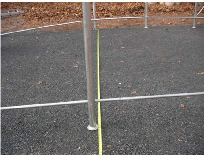
When all widths are adjusted properly, measure from diagonally from inside corner to inside corner. Adjust frame as necessary to bring frame into square. **Failure to square frame of unit will result in poor cover fit and reduced strength and rigidity.** If end or interior upright ends are placed on soft material that will not support weight, recess small patio blocks or bricks under leg ends. This will also allow better setting of frame before securing to ground.
