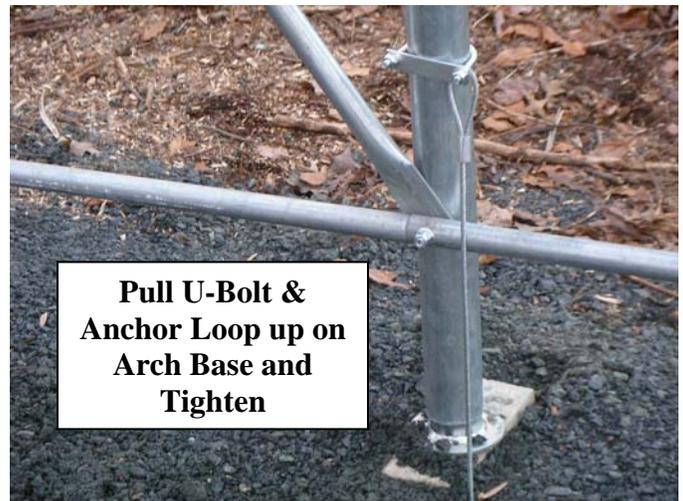
**Pull U-Bolt & Anchor Loop up on Arch Base and Tighten**
